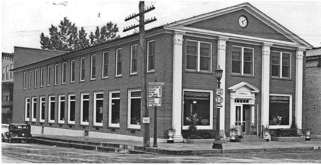
View of the former D. L. B. Smith general store after the extensive renovation work that was completed in 1936 by the Selected Risks Fire Insurance Company. PHOTO PROVIDED BY THE WANTAGE AVENUE HOLDING COMPANY
